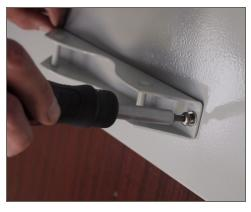
Figure 5: Attaching the banding bracket to the sign
