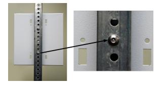
Figure 12: Pole bracket with bolts on the Telespar pole
